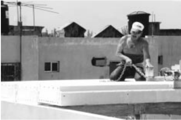
Fig. 9: Before placing the panel on the supports, remove safety chains.
