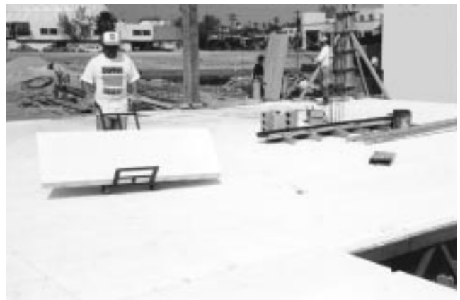
Fig. 12: Contec Slab panels on steel beams.
