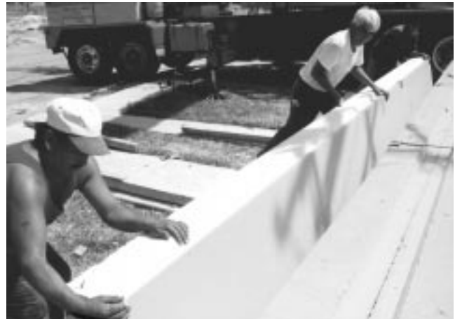
Fig. 6: Turning down the panel.
