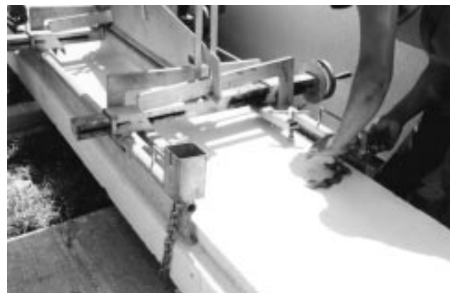
Fig. 8: Placing the lifting gear at center of panel.
