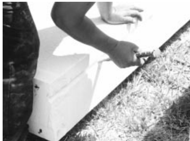
Fig. 7: Cleaning the groove side of the panel.
