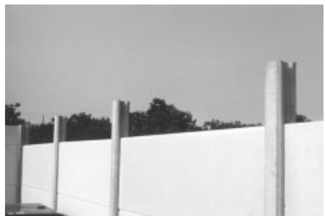
Fig. 8: Third course of Fence panels.
