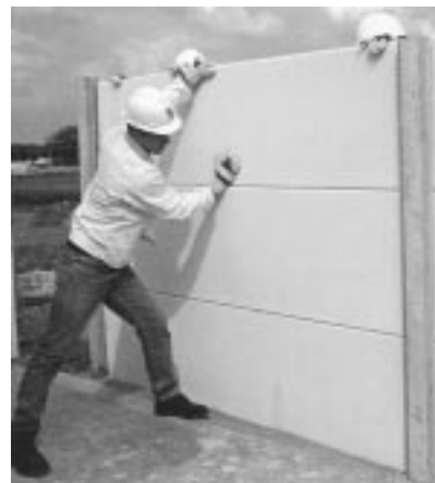
Fig. 7: Contec Fence panel installation.
