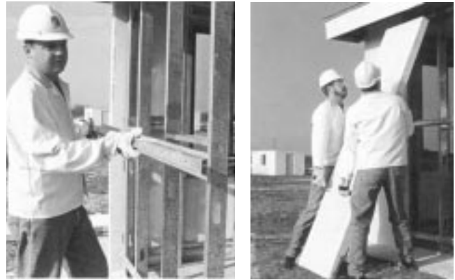
Fig. 7: Furring channel installation. Lifting Contec Board.
