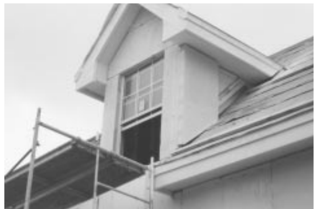
Fig. 11: Gable dormer using Contec Board.
