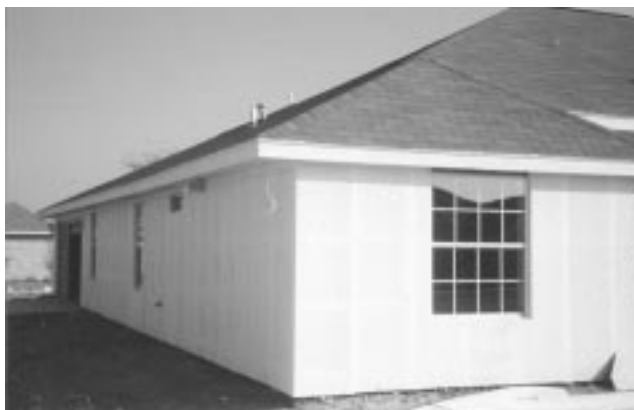
Fig. 15: Completed installation of an exterior wall using Contec Board.
