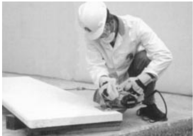
Fig. 13: Cutting Contec Board using a circular saw.
