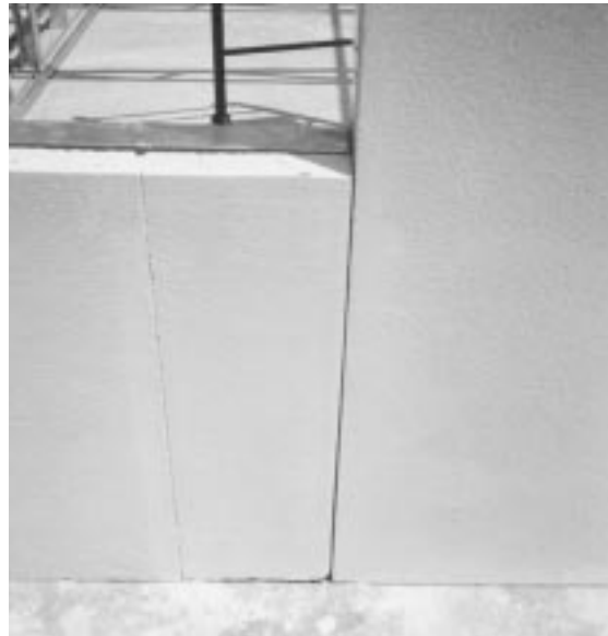
Fig. 12: Vertical control joint placed at window location.
