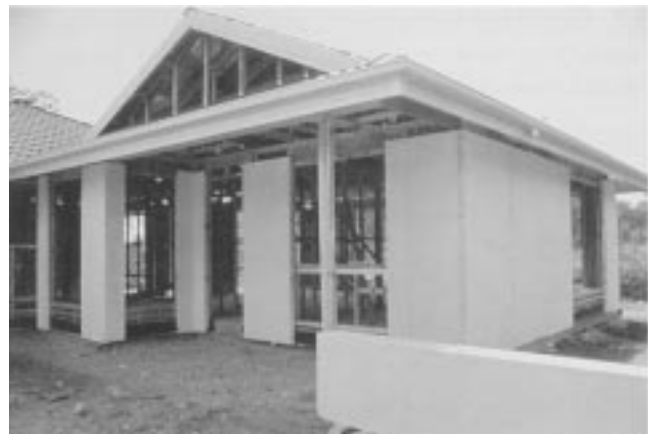
Fig. 10: It is recommended to install whole Contec boards first, and after window adjustments, etc.
