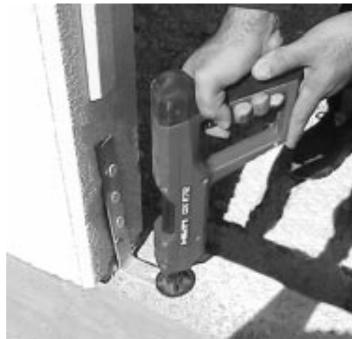
Fig. 13: Fix the lower connector (type "B" connector).
