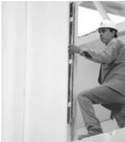
Fig. 15: Plumbing the panel in second course.
