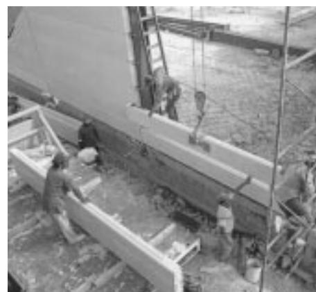
Fig. 10: Installing second panel.
