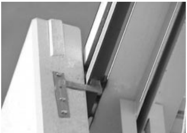
Fig. 14: Typical upper connection (type "C" connector).
