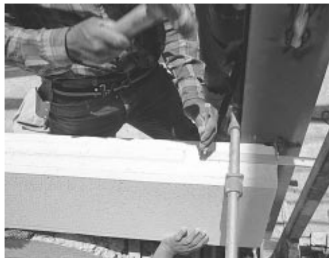
Fig. 9: Nail the connector to the panel (type A connector).
