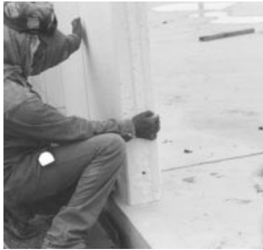
Fig. 12: Once the panel in its position, check alignment.
