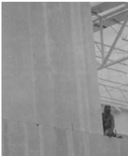
Fig. 16: Second course of Contec Vertical Wall Panels.
