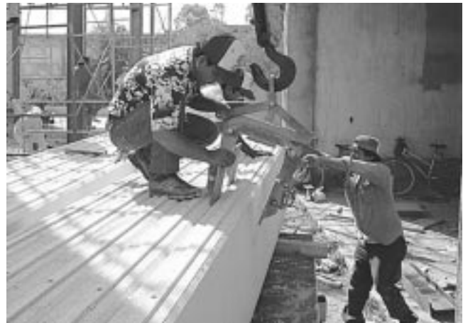
Fig. 8: Placing lifting gear at center of the panel.
