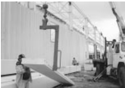
Fig. 11: Place the lifting hook into the hole and lift the panel.
